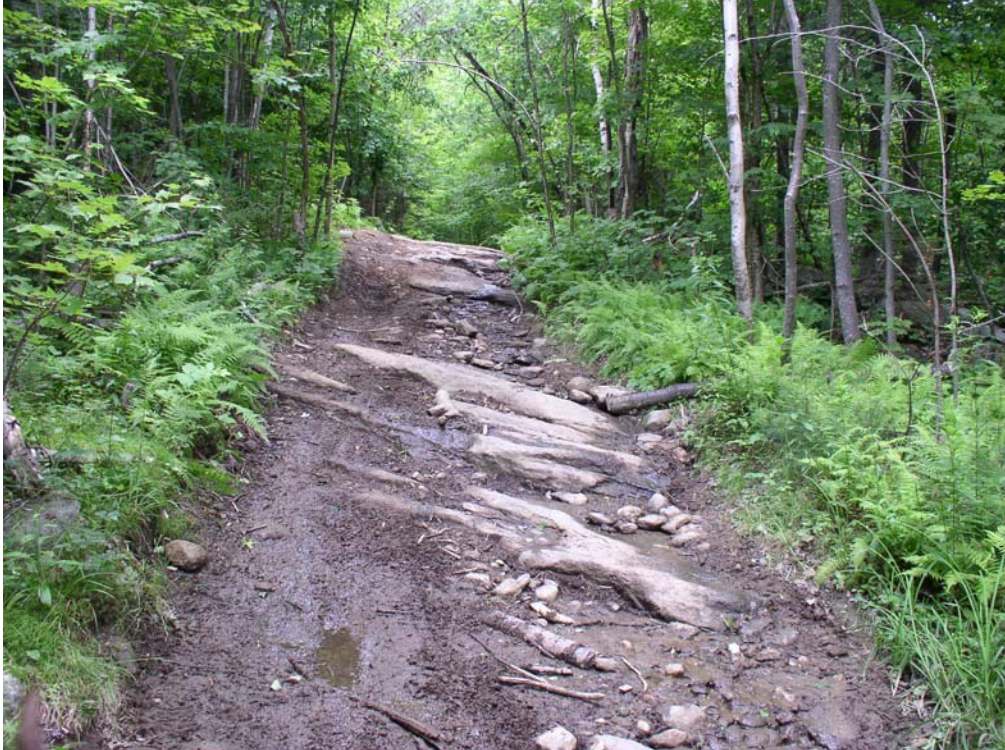
Severe erosion down to solid ledge on a steep 4WD road near Aaron's Ledge. This has changed the water drainage to follow the road, compounding the erosion.
